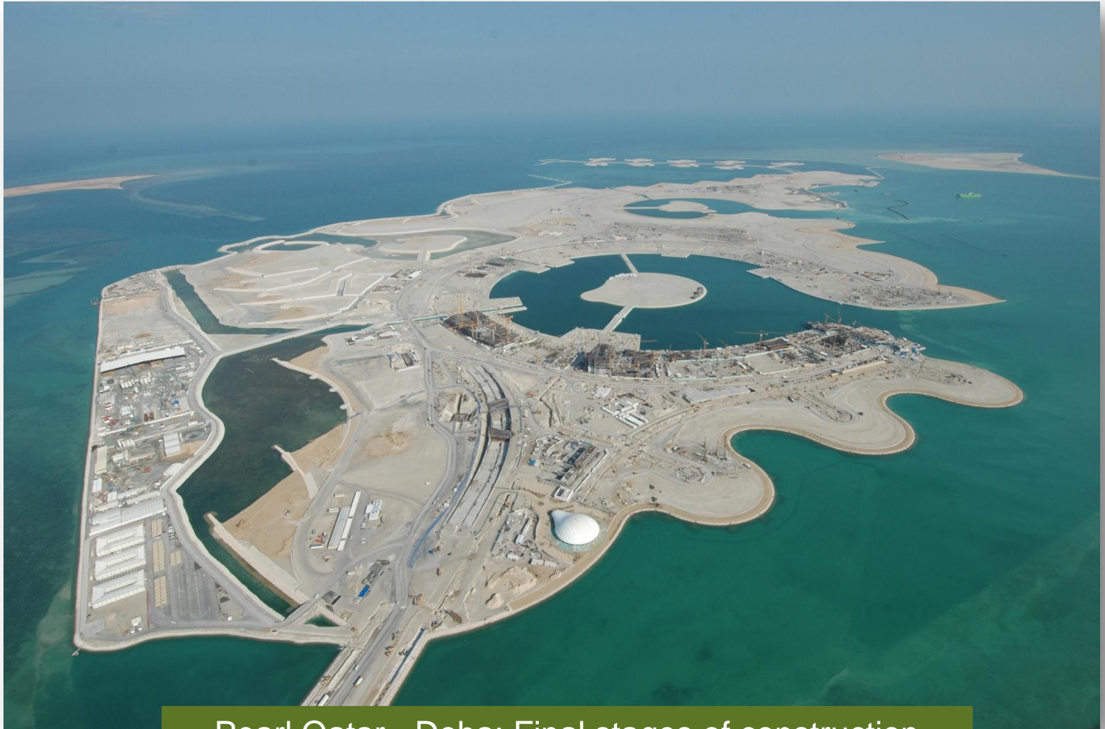
Pearl Qatar - Doha: Final stages of construction
